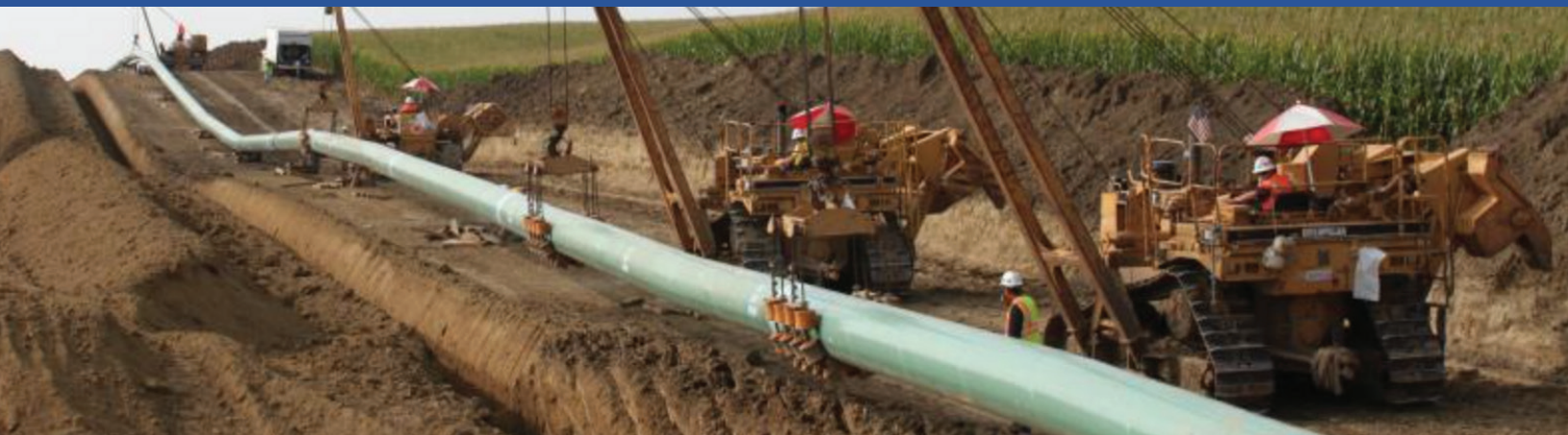
An assembled pipeline is lowered into place before the soil is replaced.
