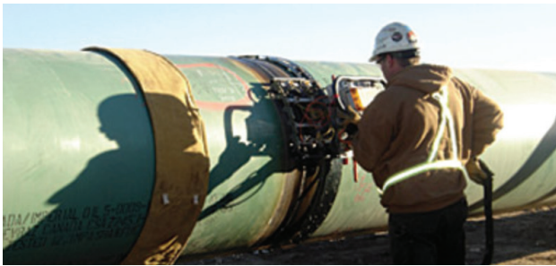
Inspection technician scanning a weld to ensure a defect free connection.
