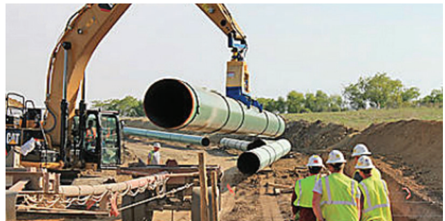
Pipe segments laid out for connection.
