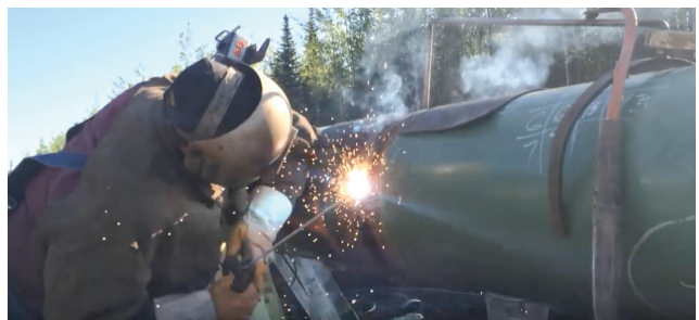
A welder joins two ends of pipe segments with a girth weld.
